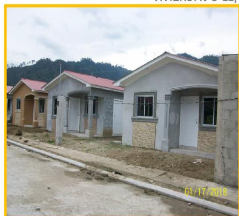
VIVIENDAS E-8, E-9, E-10 (LOTE 8)
